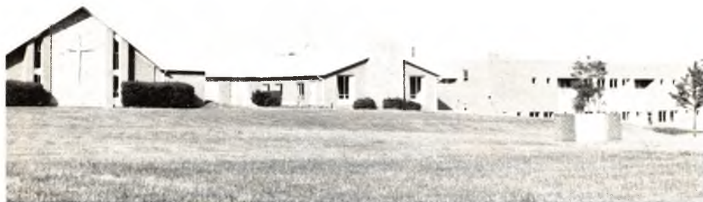
The $1.2 million family life addition of the Fairview Village Church is the largest building occupying the right half of the photo.
