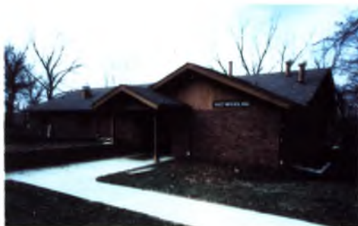
Food Service Building
