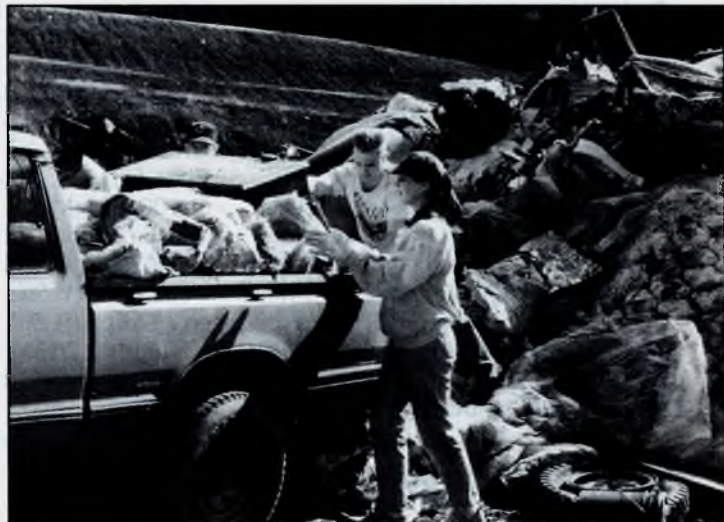
NNC students Dan Nelson, Joel Alsworth, and Robin Smith unload a truckload of damaged insulation and other items at the dump.
