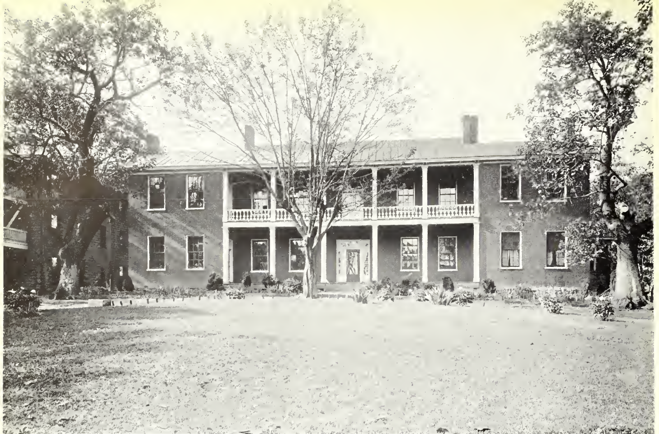
ABOVE: ADMINISTRATION BUILDING (FRONT VIEW)
